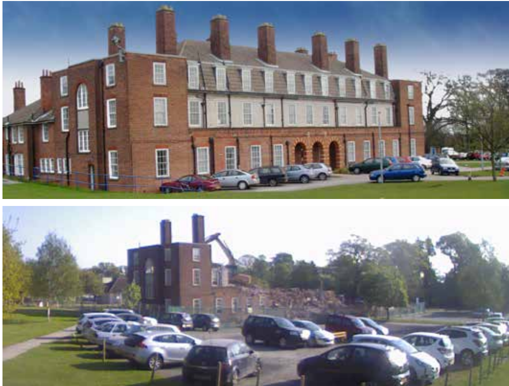
Finance Building: demolished mid 2017
