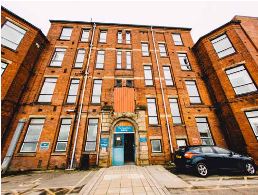
Haughton Building (West): to be demolished mid 2017
