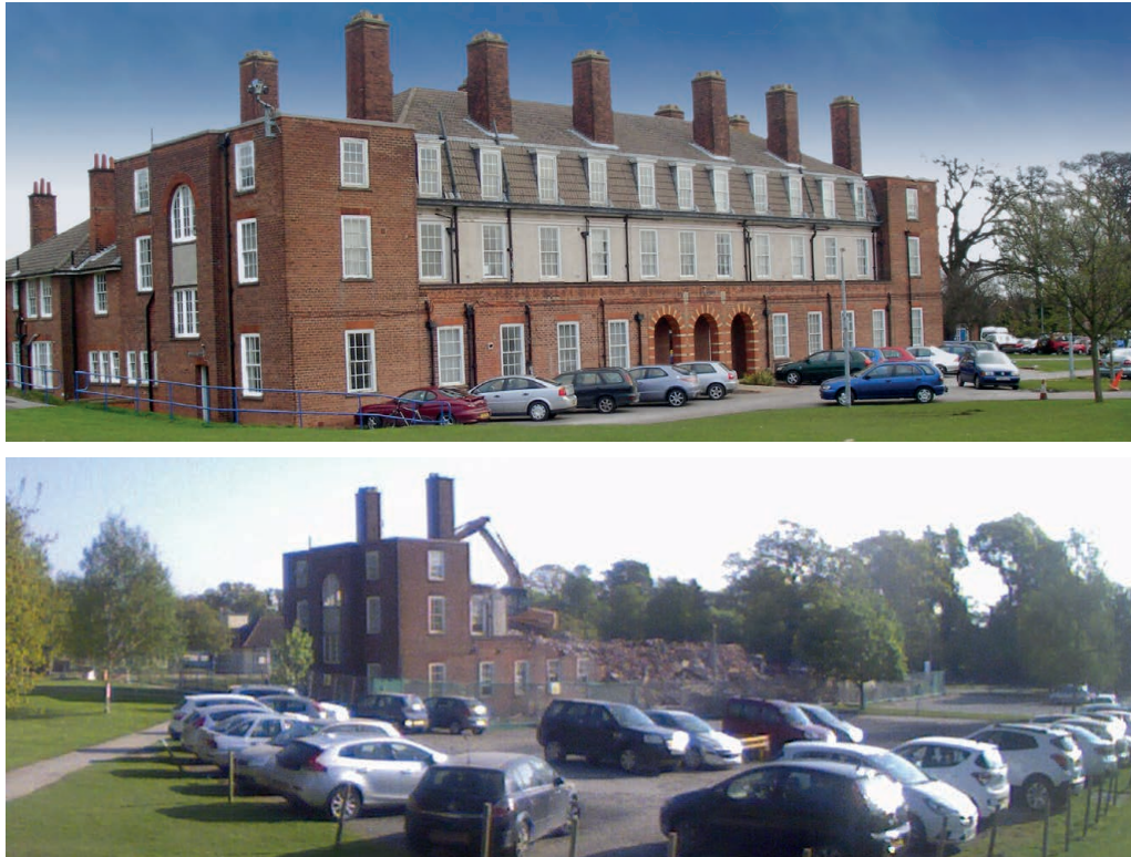
Finance Building: demolished mid 2017
